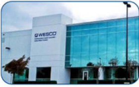
Dallas One WESCO Facility Opened 2012
