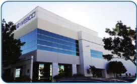
Los Angeles One WESCO Facility Opened 2013
